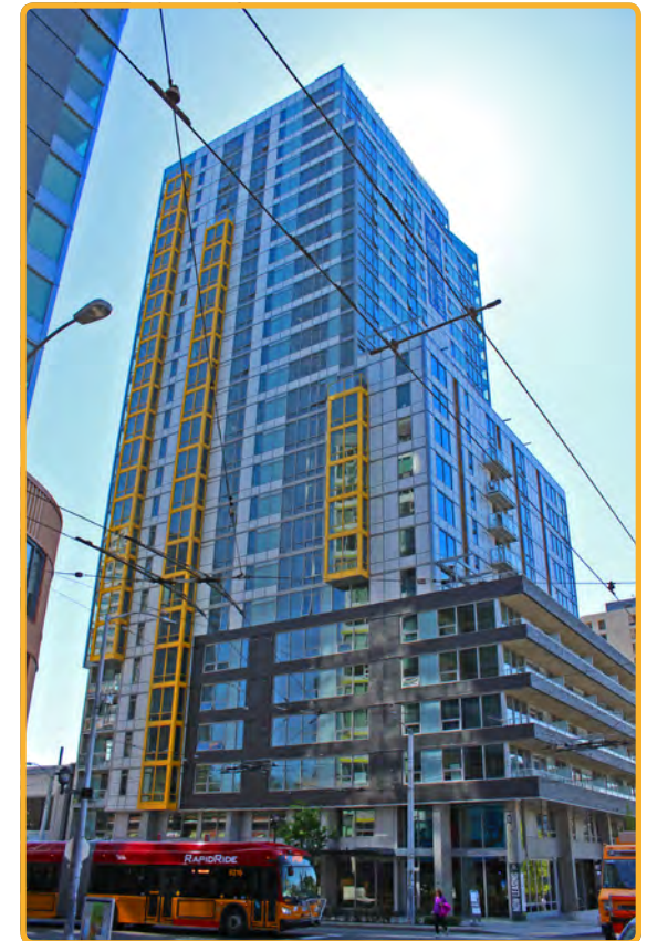
This residential tower at Cedar St and 3rd Ave in Belltown occupies roughly a quarter block and is 240 feet tall.
