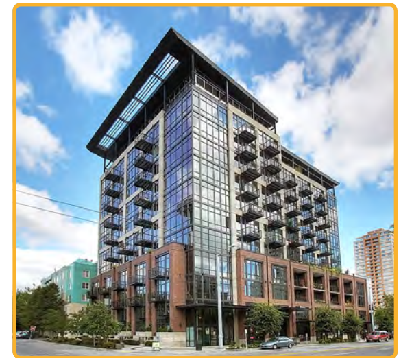
The Mosler Lofts is a 12-story residential building located at 3rd Ave between Cedar St and Clay St in Belltown.
